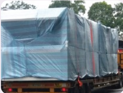
PPVC module wrapped with canvas sheets prior to delivery.
