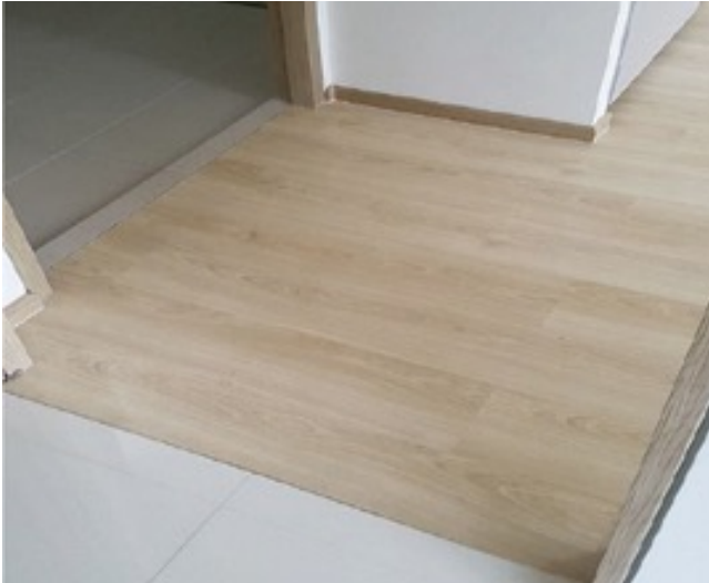
Figure 6: Use of different floor finishes to mitigate pointing alignment issues.
