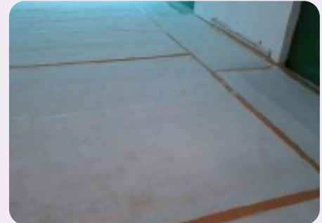
White PVC corrugated sheets for tiles/flooring protection.
