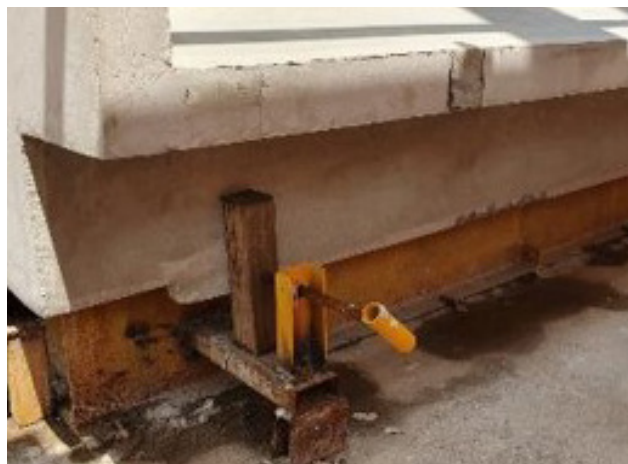
Figure 12: Adjustable props to secure the top and bottom of 2D panels.
