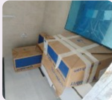
Cardboard wrapping to protect sanitary fixtures.
