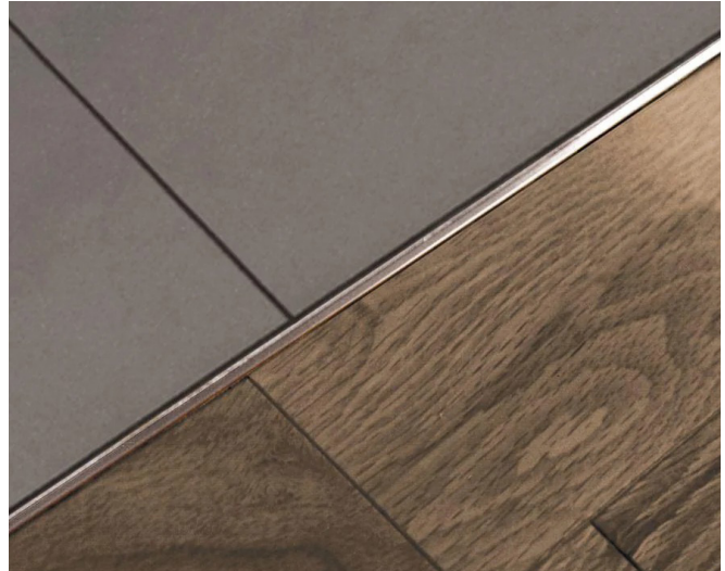
Figure 6: Use of different floor finishes to mitigate pointing alignment issues.
