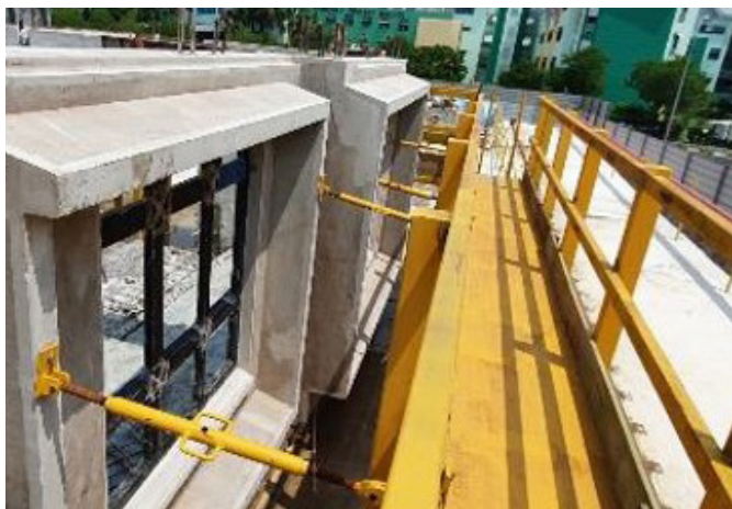
Figure 12: Adjustable props to secure the top and bottom of 2D panels.
