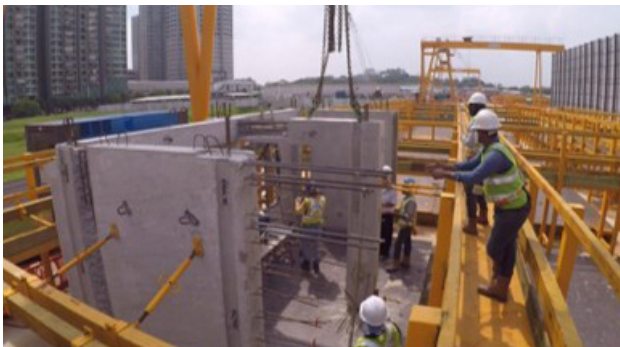
Figure 10: Use of jig/frame with adjustable props for 2D panel assembly. (Photo courtesy of Chip Eng Seng Contractors (1988) Pte Ltd)
