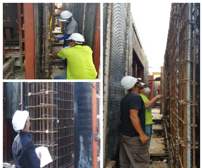
Figure 3: Inspection prior to casting.
